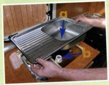
On some caravans, removing the sink will expose the fridge-top wiring. The plug hole (a) was unscrewed from the trap (b), the sink unscrewed and removed. Some have replaceable sealant.
