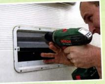
Back out of doors again, Dave, who was carrying out the work, marked the fixing positions on the fridge vent and drilled holes for the screws provided with the kit.
