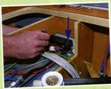
Dave unscrewed the trunking (arrowed), passed the wiring along the existing wiring route into the space atop the fridge, and used the existing foam sealant to guard against draughts.
