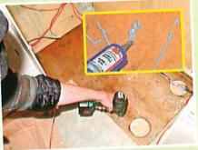
The stainless steel sheet was fixed with my old favourite, Würth Bond and Seal, and held down with screws while the sealant set.
