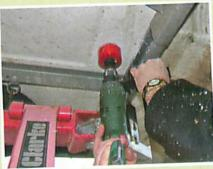
...until the centre drill just appeared below, then moved the cutter to the underfloor. The cutter size depends on the size of the waste outlet.
