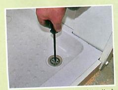
The waste outlet, with stub to attach the drain hose, is held from beneath while the grille and seal are fitted above with the central fixing screw.
