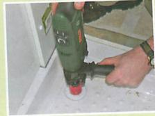
Now we could see that the drain had to be fitted to the inboard side of the shower tray so used the correct size of hole cutter from above...
