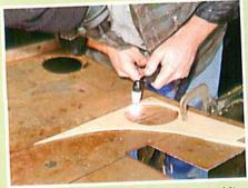
The floor flexed so we reinforced it with a steel sheet. Not yet knowing which side the drain would have to go, we cut an access hole on each side.
