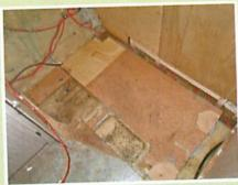
This had been a cloakroom but the floor was a peculiar shape and had to be levelled by fitting appropriately shaped pieces of marine plywood.
